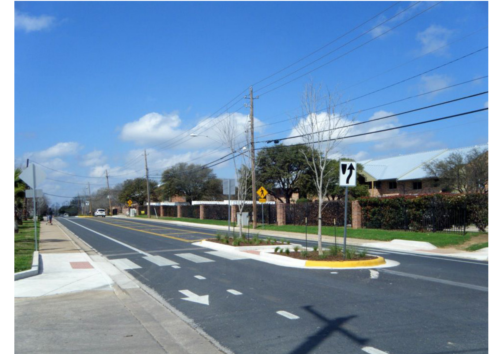
Pedestrian refuge at crossing
